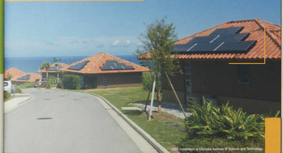
OES Installation at Okinawa Institute of Science and Technology
